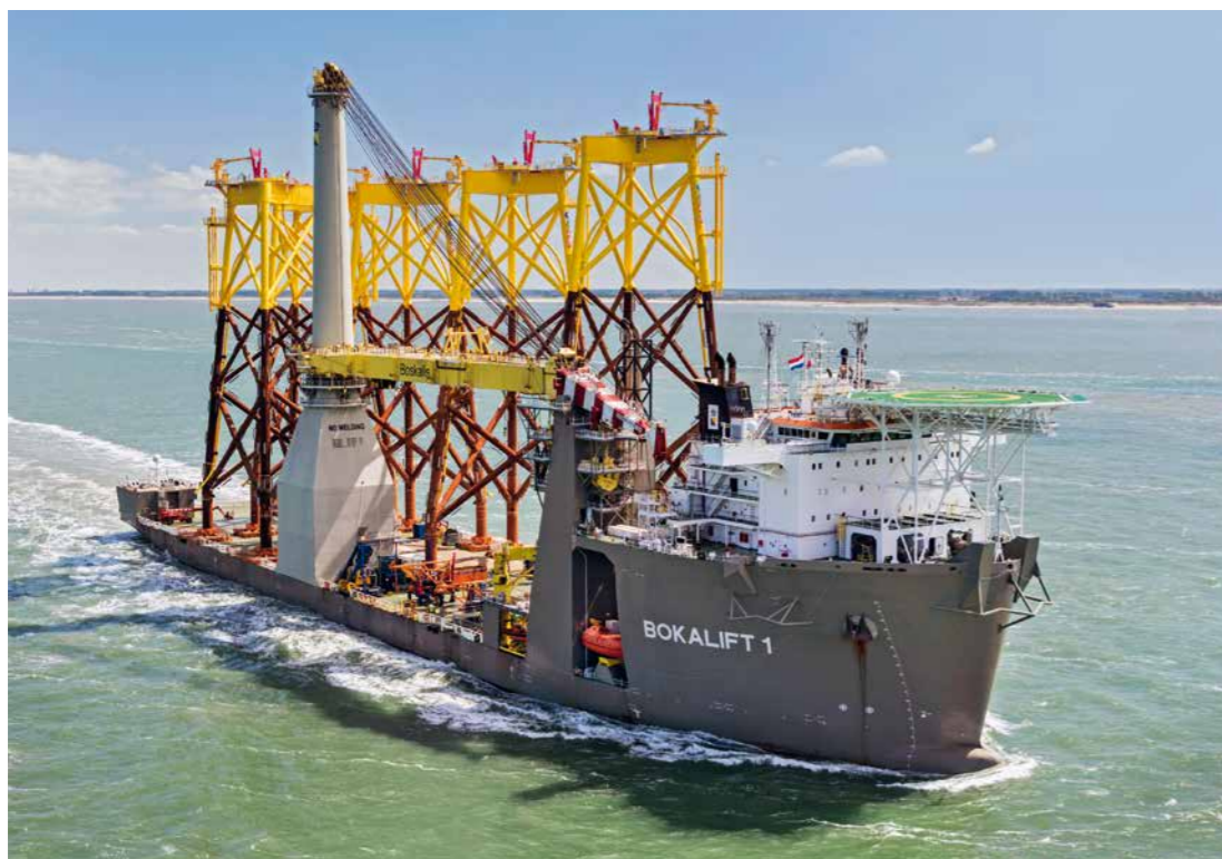
Transport and installation of jacket foundations by crane vessel Bokalift 1
