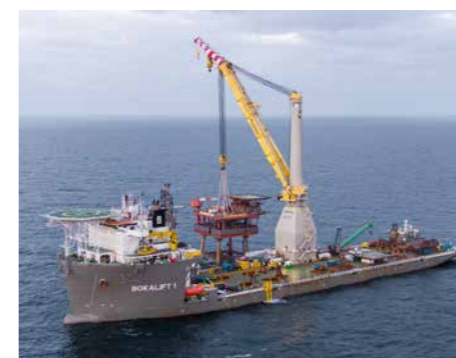
2 HEAVY LIFT VESSELS
